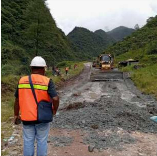
The process of revitalizing the main road access to Waa Banti village using *gravel* sand taken from the CIP 72 area of PTFI.
